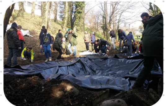
Placement of non-woven tissue on the digging carried out.
